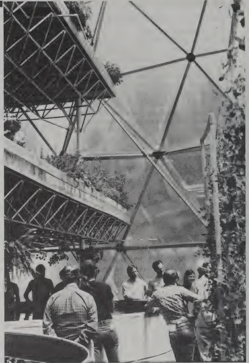
Windstar's 50 ft. Biodome at Snowmass, Colorado, grows vegetables and fish all year despite subzero winters. No fossil fuel is used; electricity comes from photovoltaic panels and a small water turbine. You can buy one, though it needs more development for use as a home. For another look at a Biodome exterior, see page 50.
